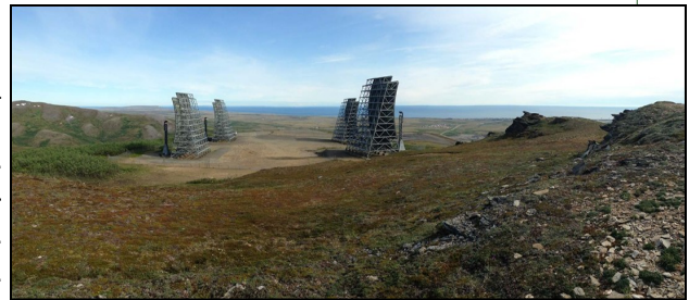
The old Cold War Troposcatter antennas still stand at the White Alice facility right outside of Nome.
