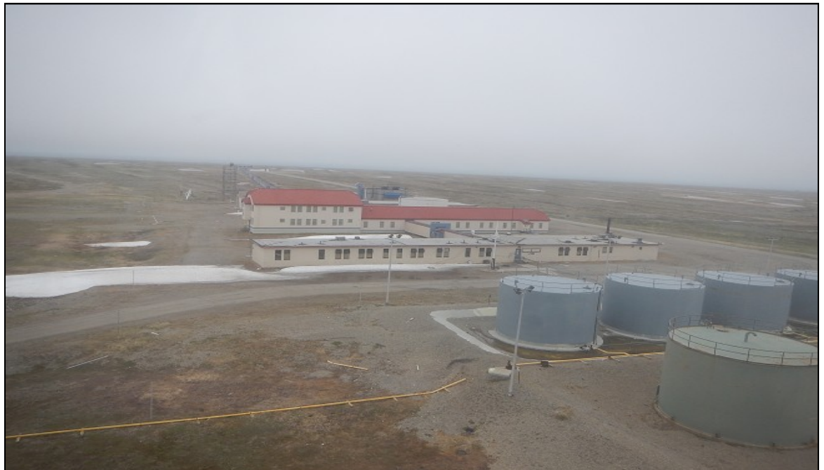
Port Clarence—Formerly manned CG LORAN station—one of our relay stations to be installed by the old transformer room. Operational concerns include interference from moose, muskox and bears. Photo by RDC Staff.
